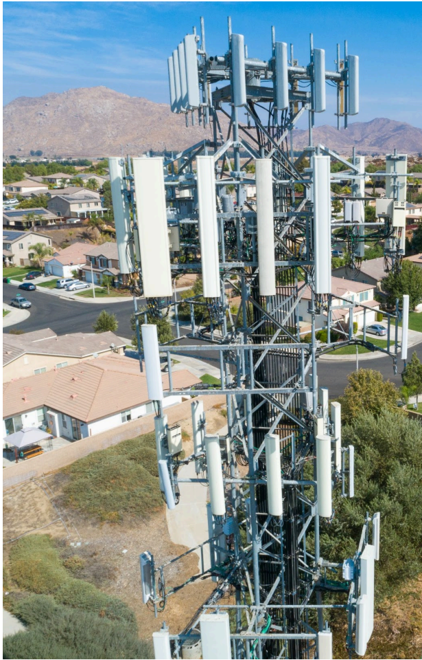
Close-up aerial of a cellular wireless mobile data tower with a neighborhood surrounding.
