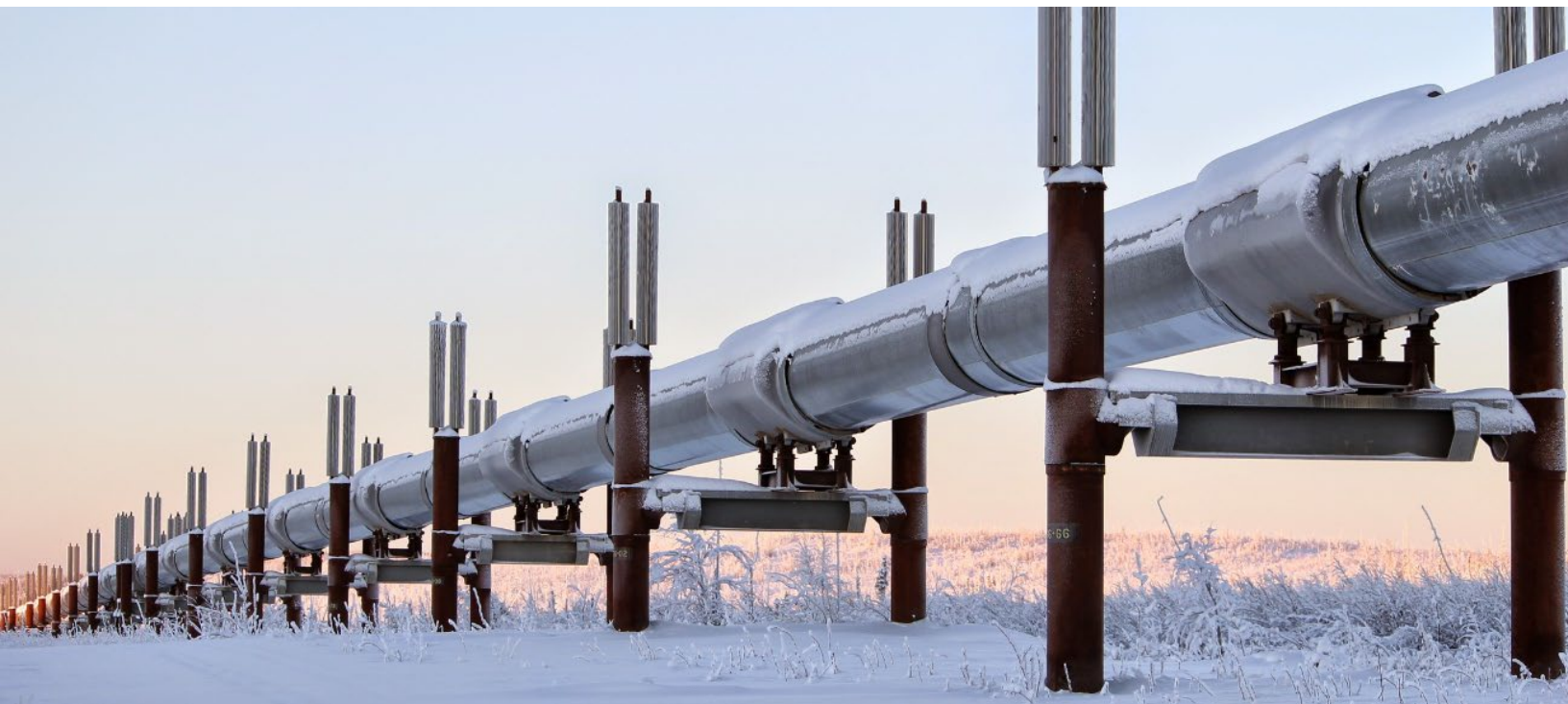
The Trans-Alaska Pipeline System.
